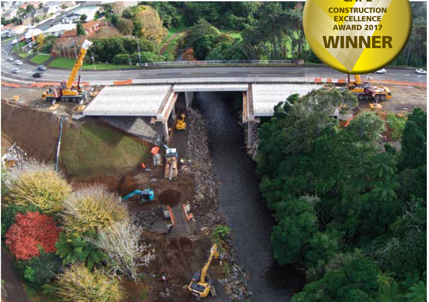
CATEGORY 2: Projects with a value of between $5 million and $20 million PROJECT: SH3 Vickers to City Upgrade. CONTRACTOR: Fulton Hogan
